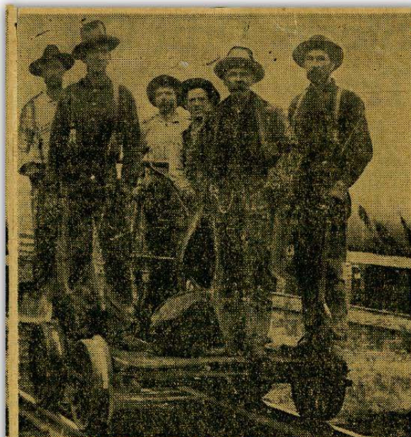
RAILROAD CREW —W. M. Ballew, second from right in this picture of a section crew on a hand car, was the first boss of the Pilot Point section of the Texas and Pacific Railroad, in 1876. Others in the picture, taken from near Pilot Point in the 'Nineties,' from left to right, are: Guy Nearrey, R. L. (Bob) Reynolds, Bill Williams, Jim Ballew and Marion Creamer.
